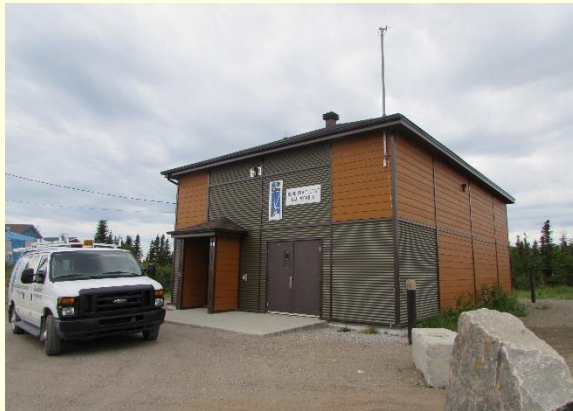
Drinking water treatment plant
